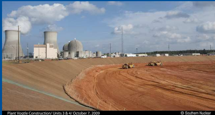
Plant Vogtle Construction/ Units 3 & 4/ October 7, 2009
