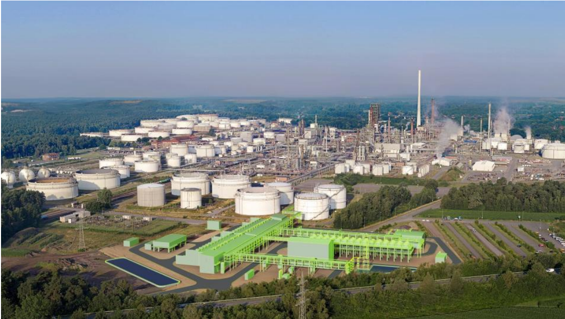
Accelera to power 100MW electrolyzer system for bp's Lingen green hydrogen project
