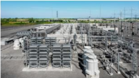
Static Var Compensator (SVC)
