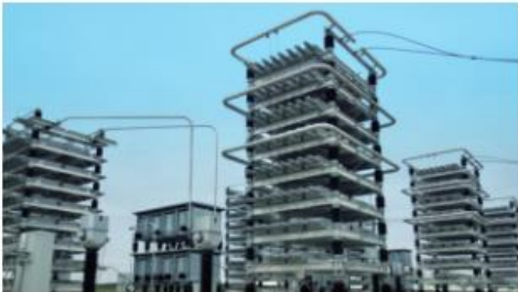
Mechanically Switched Capacitors / Filter Circuits
