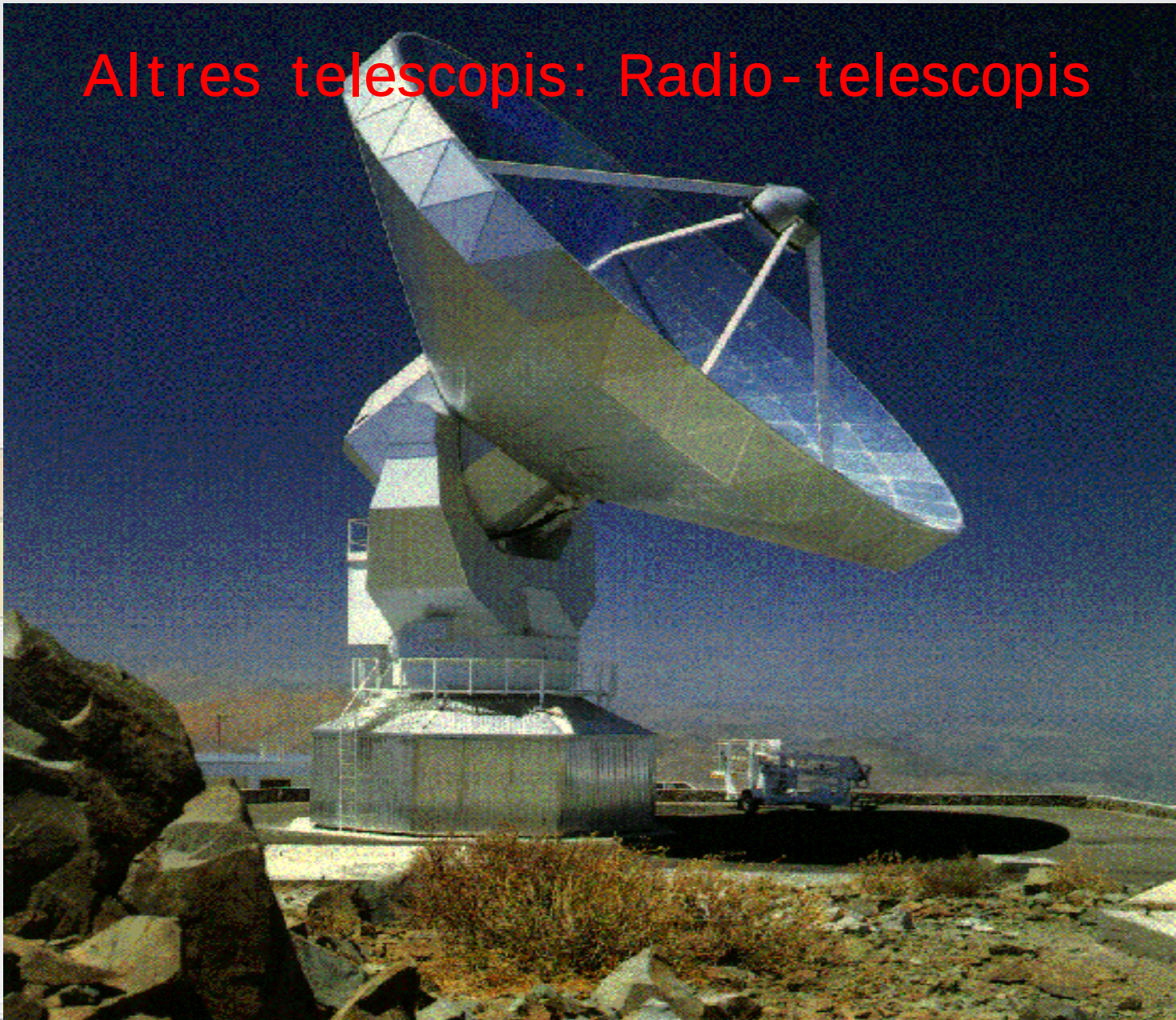
SEST: Diametre 15 m 84 GHz - 147 GHz - La Silla, Chile
