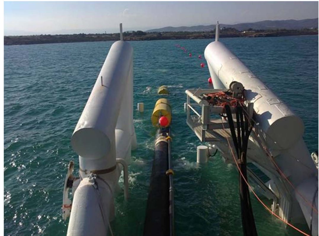
Pipeline laying (S-355 stinger)
